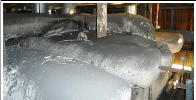
Photo 21: Insulation covered by refractory cement / POP to make the boiler roof leak proof.
