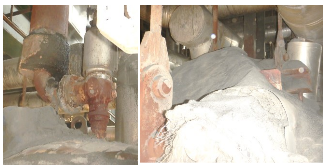
Photo 19 & 20: Uninsulated vent valve & well insulated thermowell.
