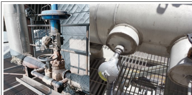
Photo 17 & 18: Uninsulated vent valve & well insulated thermowell.
