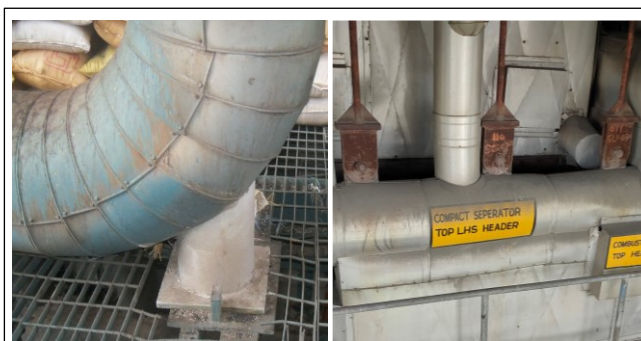
Photo 15 & 16 : Insulation to cover the attachments made to the thick walled pipes / headers
